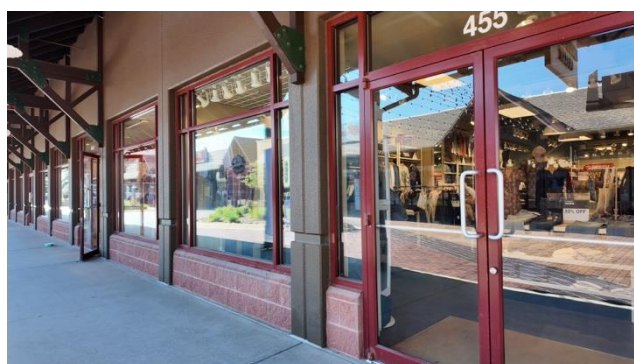
Outlets at Castle Rock
