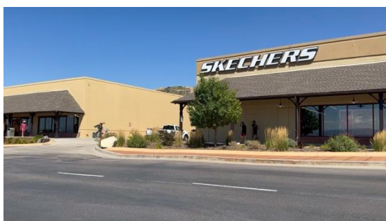
Outlets at Castle Rock
